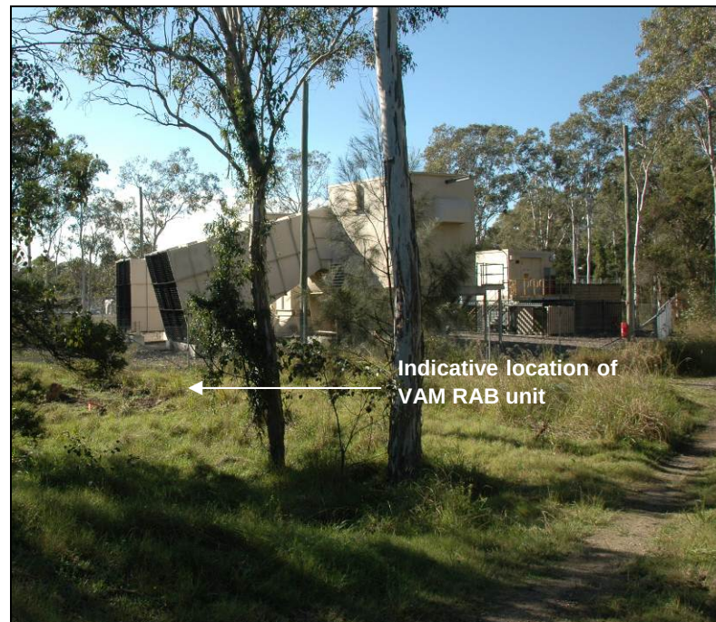
Plate 7 – Main mine ventilation fans and indicative location of VAM RAB unit
